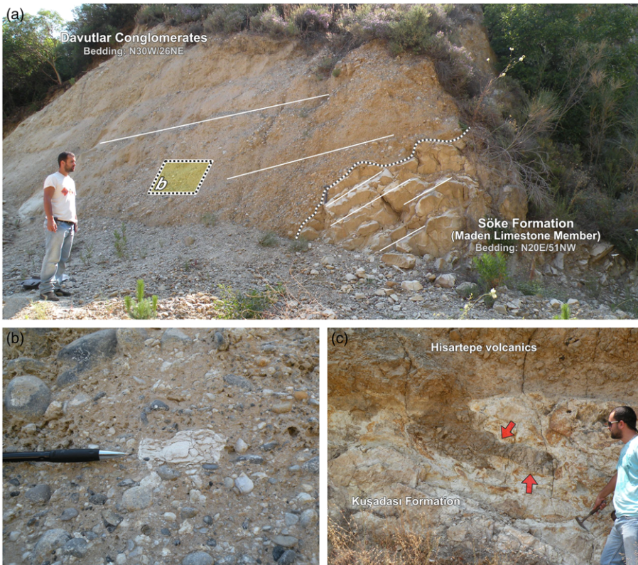
Fig. 4. Field photographs showing contact relations of the Miocene units. (a) Angular unconformity between the Maden Limestone Member of the Söke Formation and the Davutlar Conglomerate (the continuous white lines indicate bedding of the units; the bold dotted curve indicates the trace of angular unconformity); (b) angular clayey limestone clast observed in the Davutlar Conglomerate derived from Maden Limestone Member; (c) peperitic contact, arrows show the fluidal margin between a lava flow of the Hisartepe volcanic series and the limestone of the Kuşadası Formation (pen 14 cm; person 190 cm).
