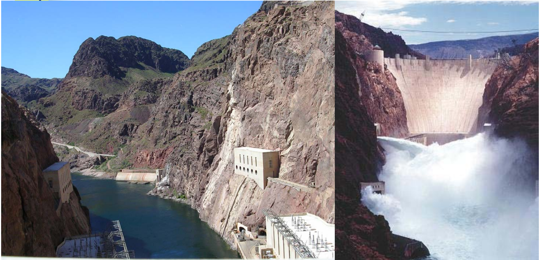
Hoover Dam Outlets
