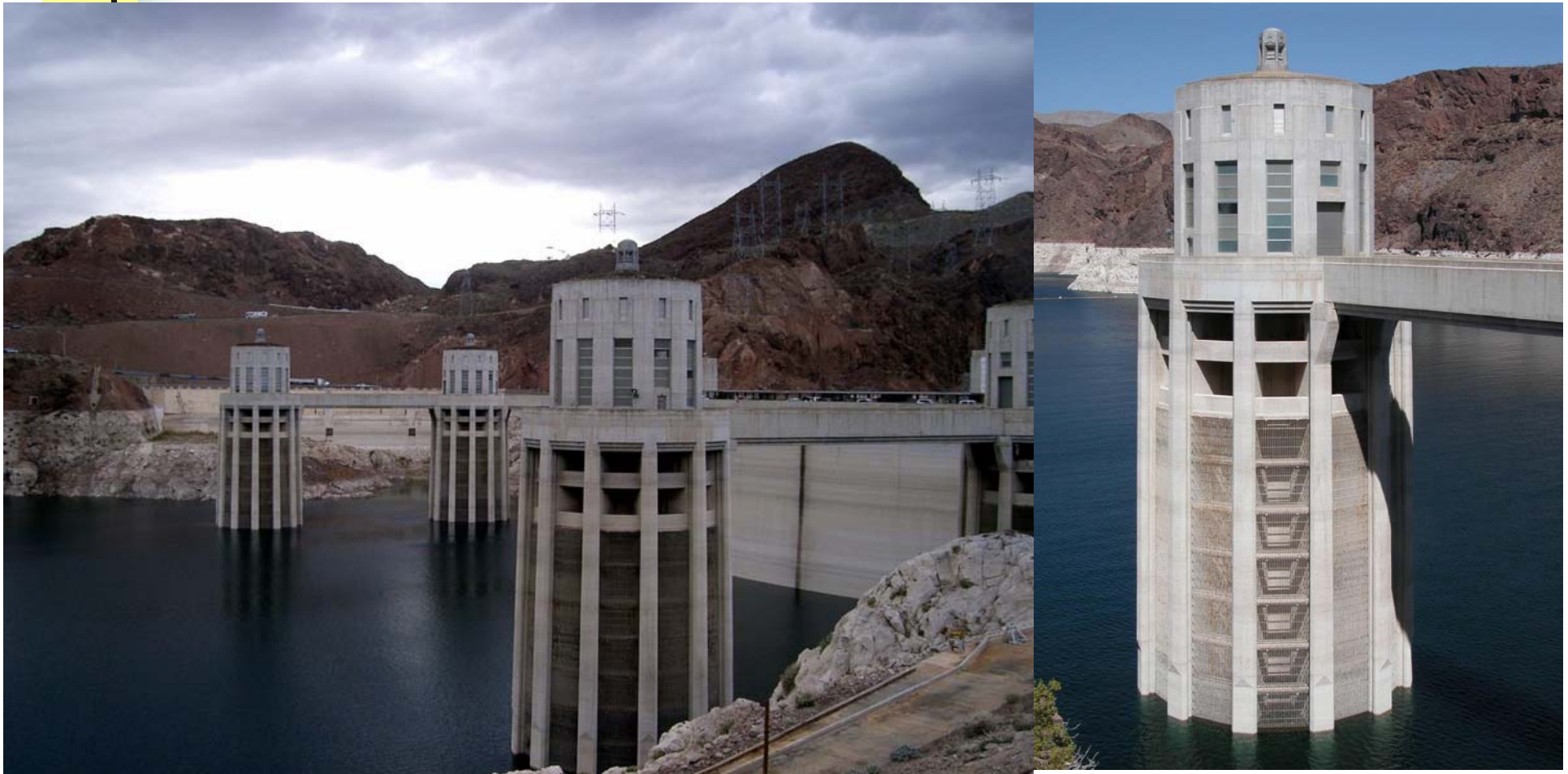
Hoover Dam Inlets
