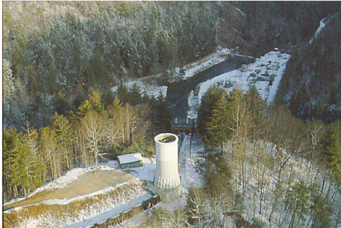
Tuxedo Dam penstock (l), surge tank (c), and powerhouse (mid-center), Green River
